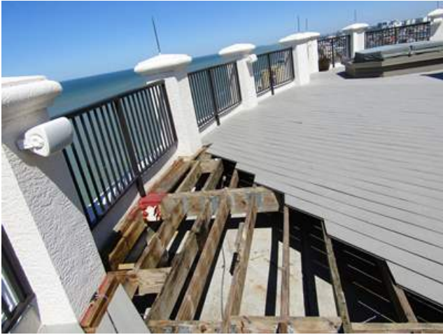
View of the roof system below a PH terrace
