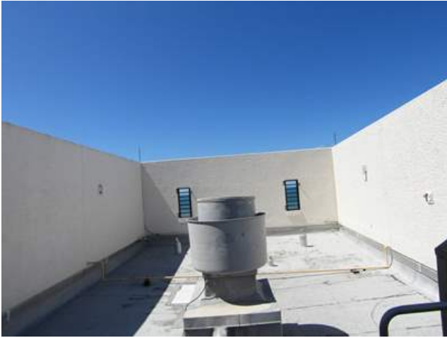
View of modified bitumen roofing system
