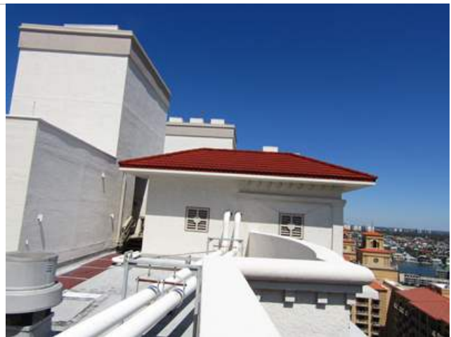
View of metal panel roof system.
