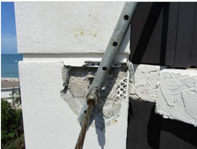
PT cable repair
