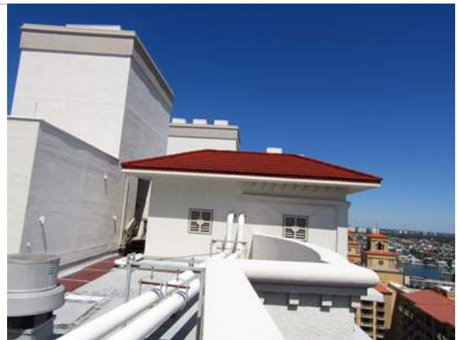
View of metal panel roof system.
