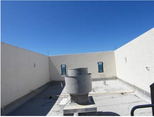
View of modified bitumen roofing system
