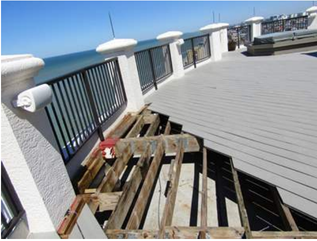
View of the roof system below a PH terrace
